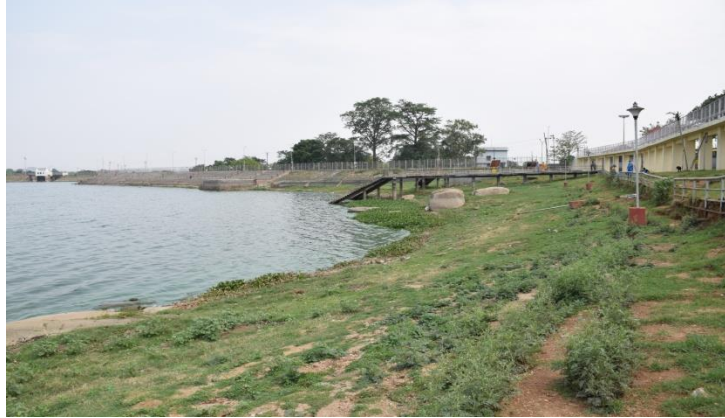
Kanke Dam after Cleaning
